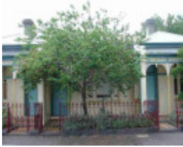
carlton north station street carlton north station street 212
