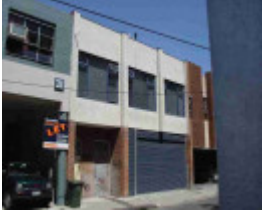
richmond wangaratta street richmond wangaratta street 23
