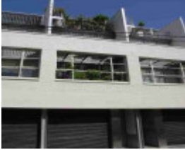
richmond wangaratta street richmond wangaratta street 24
