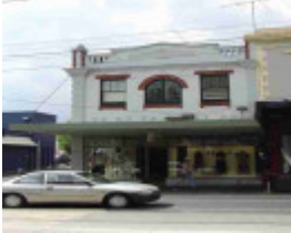
richmond swan street richmond swan street 173a
