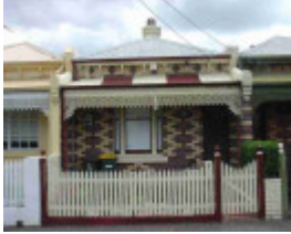
carlton north station street carlton north station street 627
