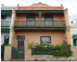
carlton north station street carlton north station street 628
