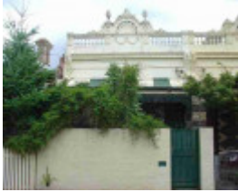
carlton north station street carlton north station street 665
