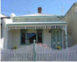
clifton hill aitken street clifton hill aitken street 15
