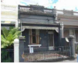
carlton north station street carlton north station street 519
