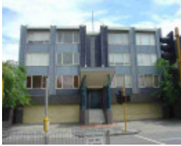
carlton north nicholson street carlton north nicholson street 427-437
