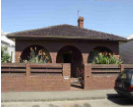
burnley queen street burnley queen street 6
