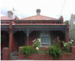
carlton north station street carlton north station street 557
