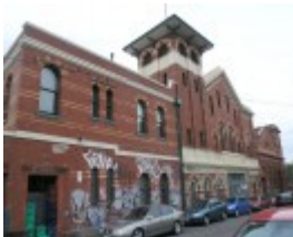
FORMER RICHMOND POWER STATION SOHE 2008
