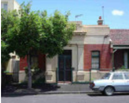
richmond stanley street richmond stanley street 18a
