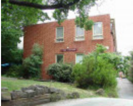
richmond the vaucluse richmond the vaucluse 2
