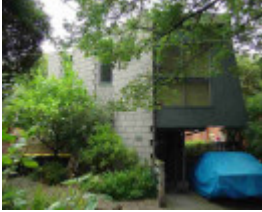
richmond the vaucluse richmond the vaucluse 4
