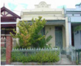
carlton north station street carlton north station street 475
