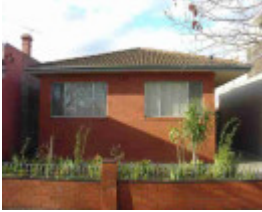
clifton hill fenwick street clifton hill fenwick street 68
