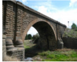
RAIL BRIDGE SOHE 2008
