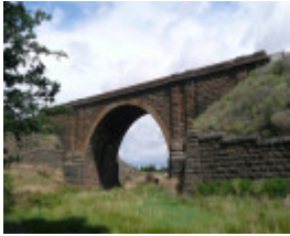
RAIL BRIDGE SOHE 2008
