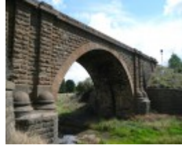
RAIL BRIDGE SOHE 2008
