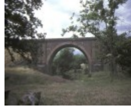
1 rail bridge over riddells creek side view dec1984
