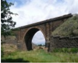
RAIL BRIDGE SOHE 2008
