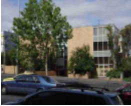
richmond punt road richmond punt road 195-199
