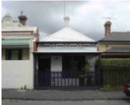
richmond the crofts richmond the crofts 22
