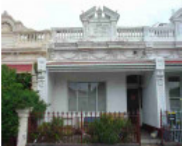
carlton north richardson street carlton north richardson street 85
