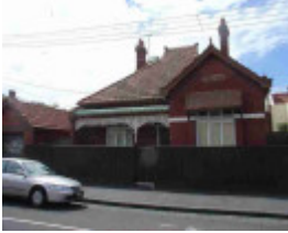
carlton north richardson street carlton north richardson street 86
