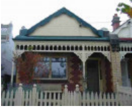
clifton hill heidelberg road clifton hill heidelberg road 21
