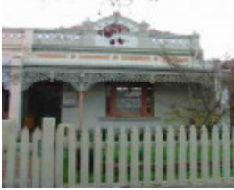
clifton hill heidelberg road clifton hill heidelberg road 23
