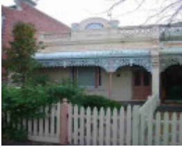
clifton hill heidelberg road clifton hill heidelberg road 25
