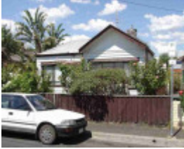
richmond wangaratta street richmond wangaratta street 5
