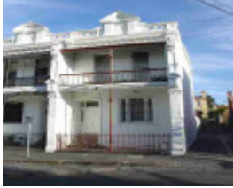
fitzroy moor street fitzroy moor street 10
