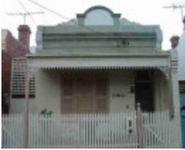
fitzroy north coleman street fitzroy north coleman street 30
