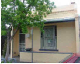
fitzroy north coleman street fitzroy north coleman street 32
