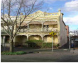
fitzroy napier street fitzroy napier street 266
