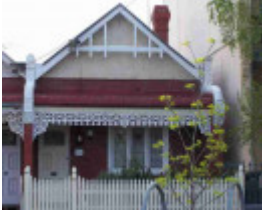
fitzroy north bennett street fitzroy north bennett street 45
