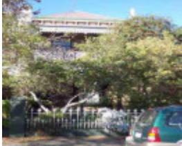
fitzroy north bennett street fitzroy north bennett street 46
