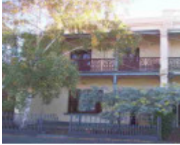
fitzroy north bennett street fitzroy north bennett street 47
