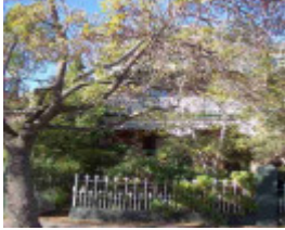
fitzroy north bennett street fitzroy north bennett street 48
