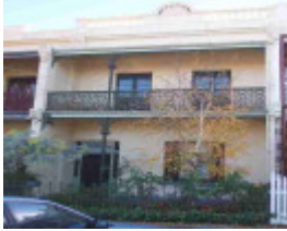
fitzroy north bennett street fitzroy north bennett street 49
