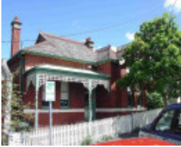
richmond docker street richmond docker street 48
