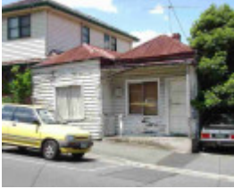
richmond docker street richmond docker street 51
