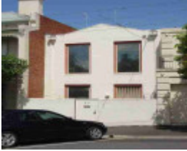
richmond docker street richmond docker street 54
