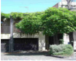
richmond docker street richmond docker street 66
