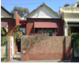
fitzroy north bennett street fitzroy north bennett street 17
