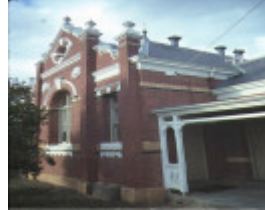
1 rochester court house rochester front elevation jul1984
