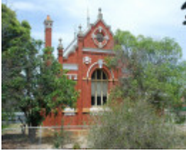
ROCHESTER COURT HOUSE SOHE 2008
