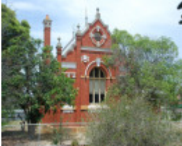
ROCHESTER COURT HOUSE SOHE 2008
