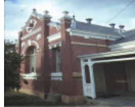
1 rochester court house rochester front elevation jul1984
