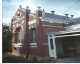
1 rochester court house rochester front elevation jul1984
