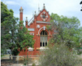
ROCHESTER COURT HOUSE SOHE 2008
