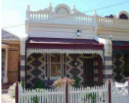
fitzroy north bennett street fitzroy north bennett street 18
