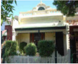
fitzroy north bennett street fitzroy north bennett street 19
