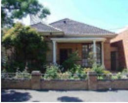
fitzroy north bennett street fitzroy north bennett street 20
