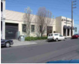
fitzroy kerr street fitzroy kerr street 190-196
