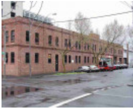
fitzroy kerr street fitzroy kerr street 221
