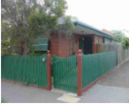
fitzroy north holden street fitzroy north holden street 40
