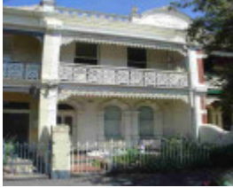
fitzroy north church street fitzroy north church street 28
