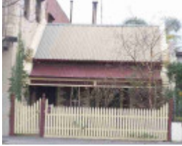
fitzroy north nicholson street fitzroy north nicholson street 422
